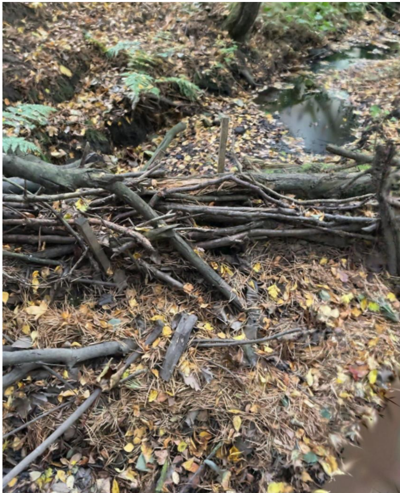
A 3D scan of a leaky dam in Stanley Burn, South Moor captured using Scaniverse
