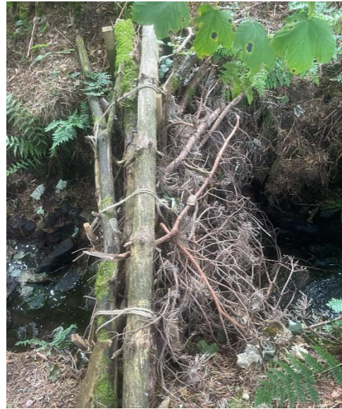
Figure 9 – Photographs to capture the different types of dam. A). Natural woody debris dam, with loosely placed long branches and other fallen material across the channel B). Wooden-Boarded Dam, created by cutting a groove into either bank side and using several plank-like pieces of wood C). Geotextile-assisted dam using rope and wooden pegs to hold it in place (Classifications adapted from Hansamali et al., 2025).
