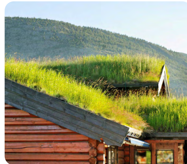
SuDS Green roof | Ratikova
